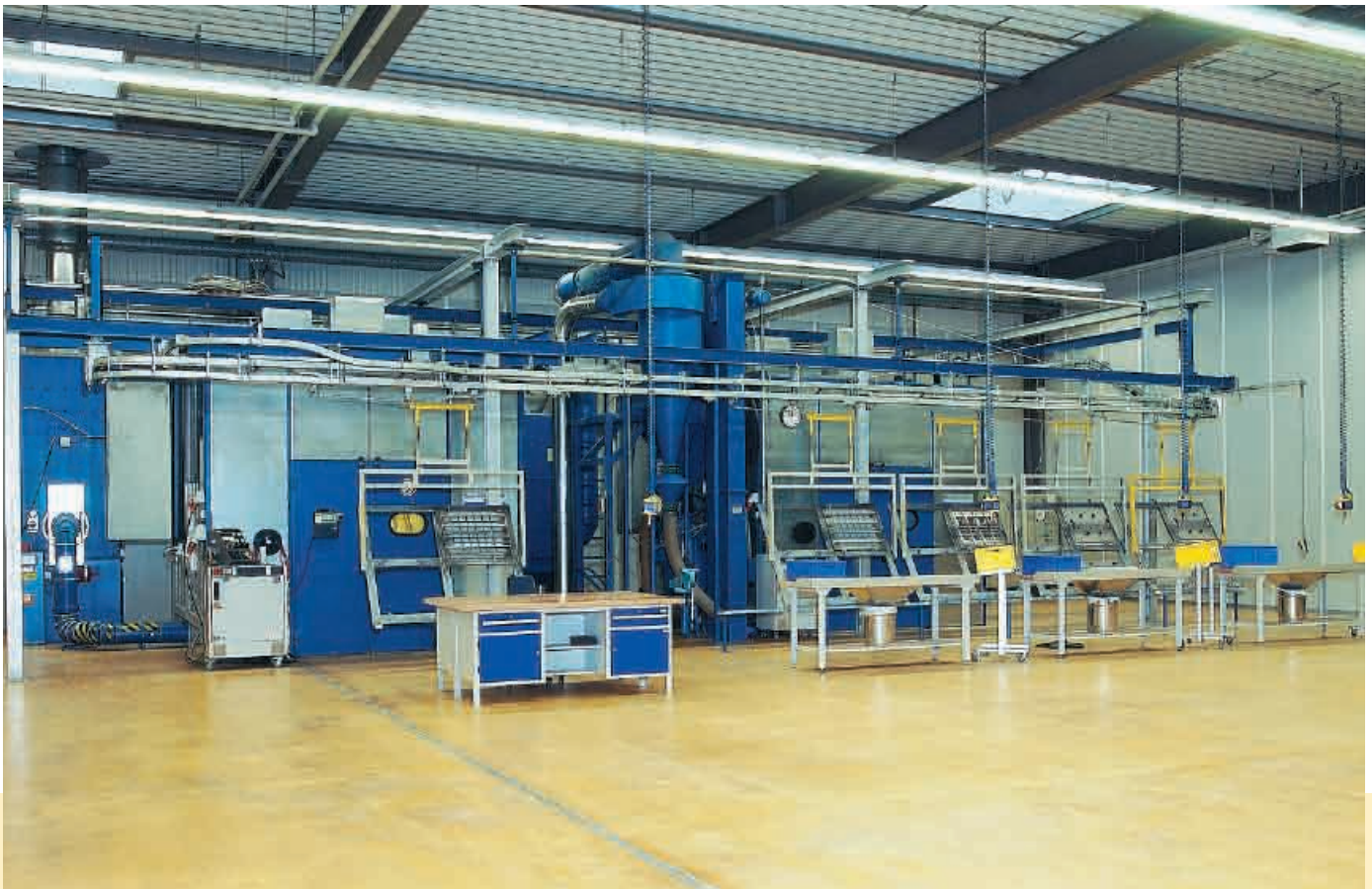
Coating production plant
